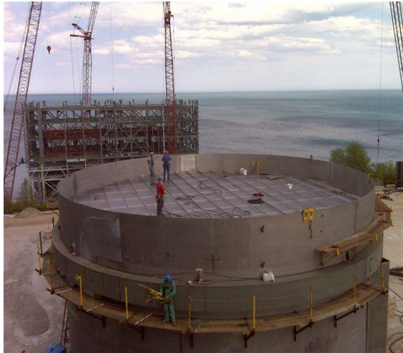
Figure 3 – DFT used as Staging Platform during Construction
