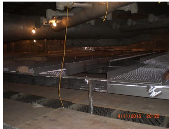
Figure 5 – 2 nd layer DFT addition
