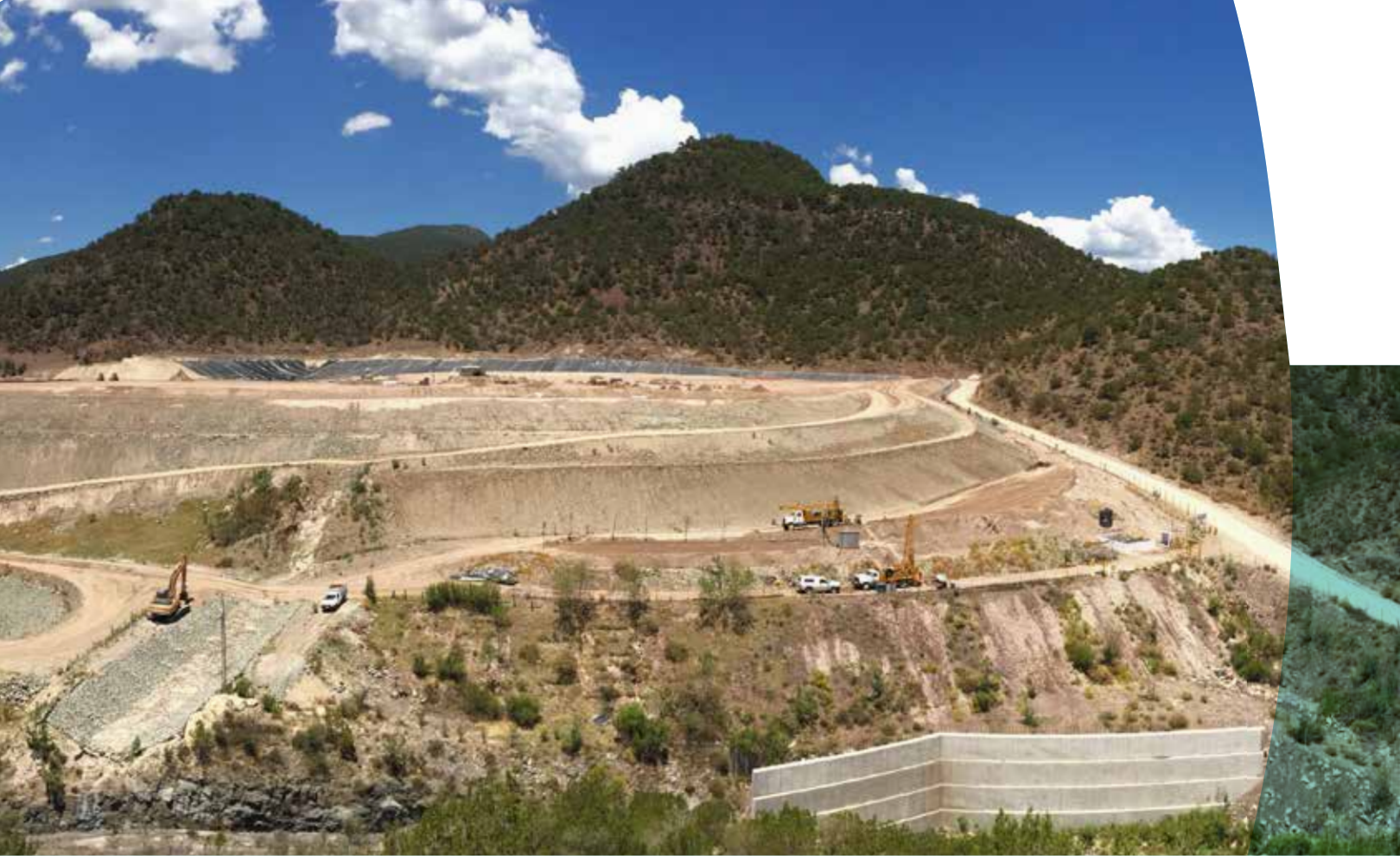
Mina Guanaceví, Endeavour Silver Corp.
